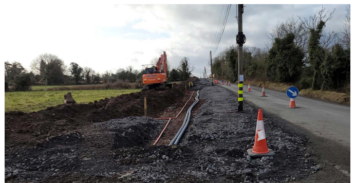
Roads laying of ducting for Ennybegs Active Travel Project
